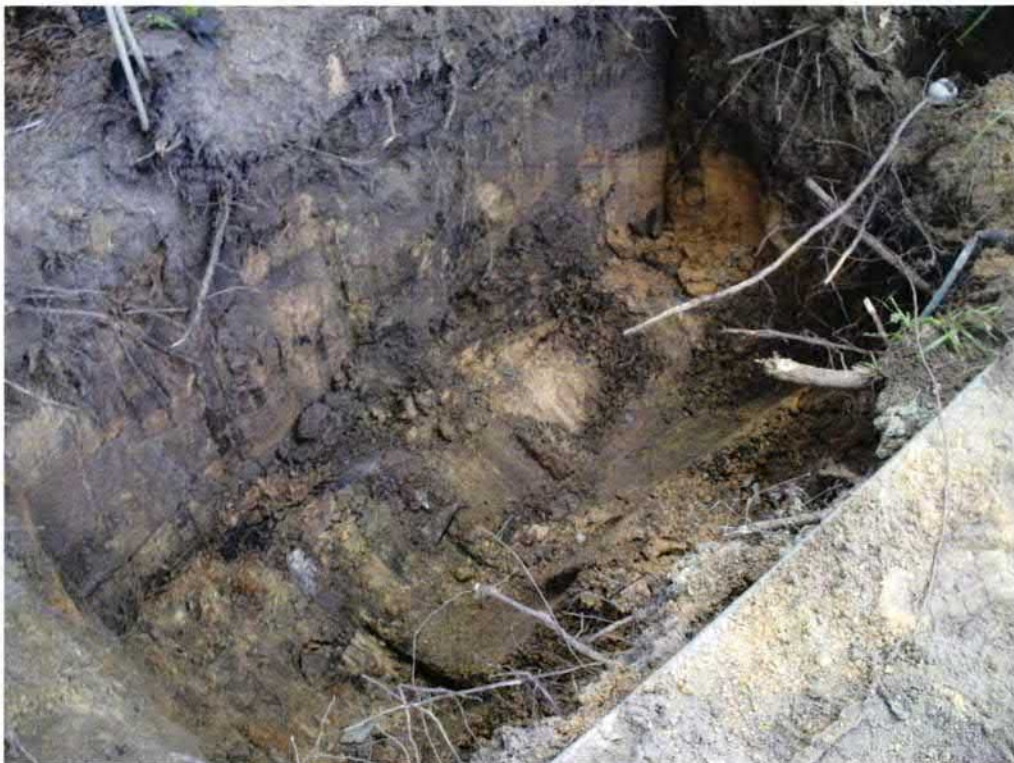
Picture 2: UST 683Camellia excavation after tank removed.
